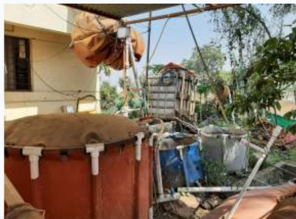
Low-cost biogas plant that gives slurry which, when filtered and mixed with water, can be used as water soluble fertiliser (given through drip irrigation network)
