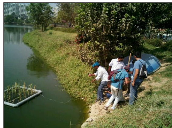
Floating island being installed at Kaikondrahalli lake (2017) [Photo Credit: Biome]
