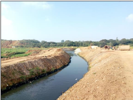
Temporary diversion channel carrying stormwater and wastewater away from Bellandur lake towards Varthur, 2020 [Photo Credit: Sumita Bhattacharya]
