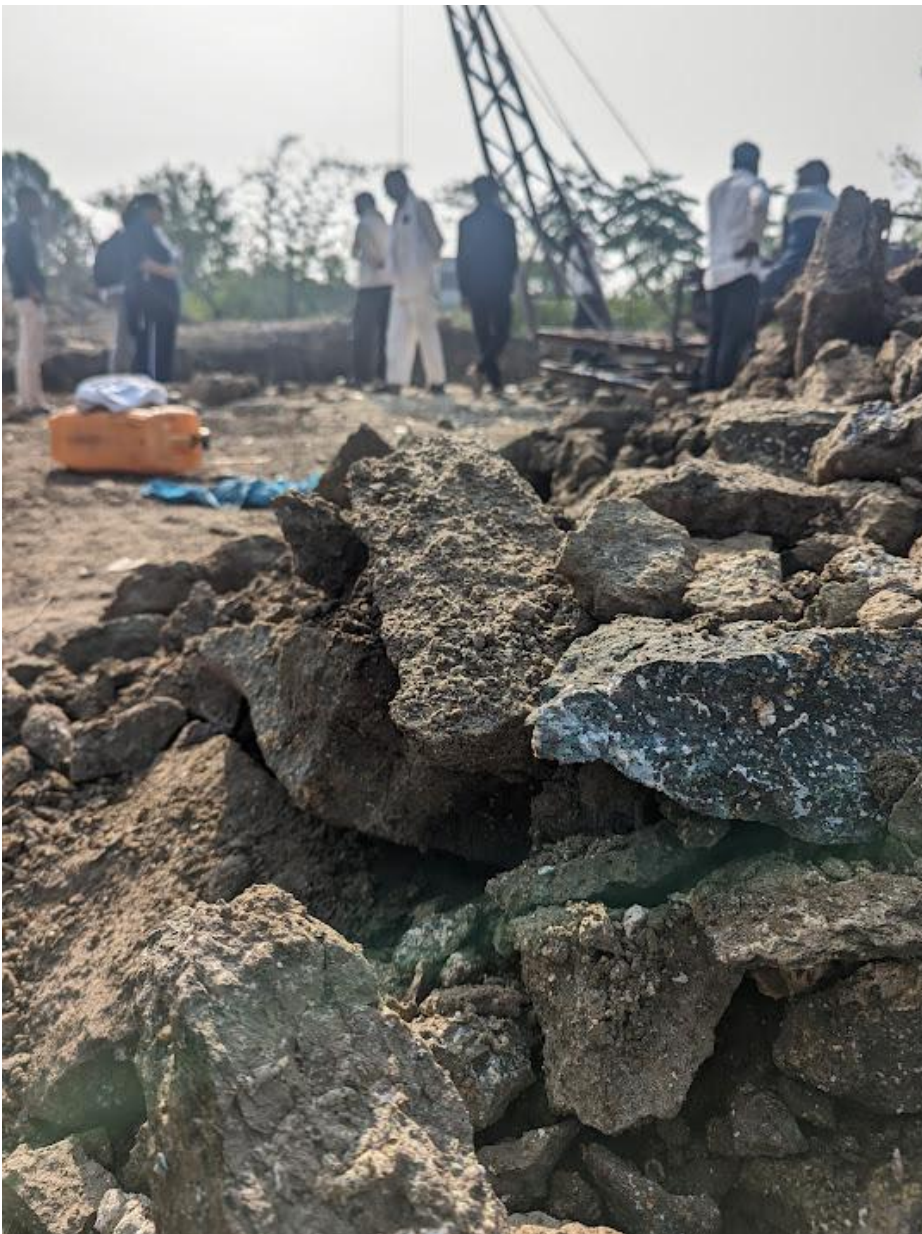
Figure 3: Boulders excavated from a well, to be used to fill a JalTara pit. Credit: Vivek Grewal
