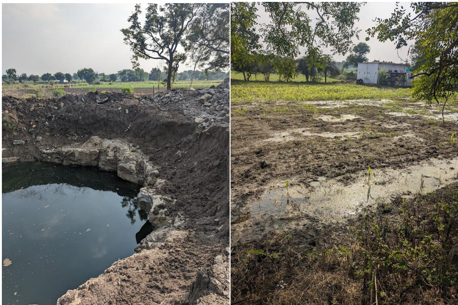
Figure 33a (left): A well being dug; these boulders are used to fill JalTaras. Figure 33b (right): Waterlogging in a field.
