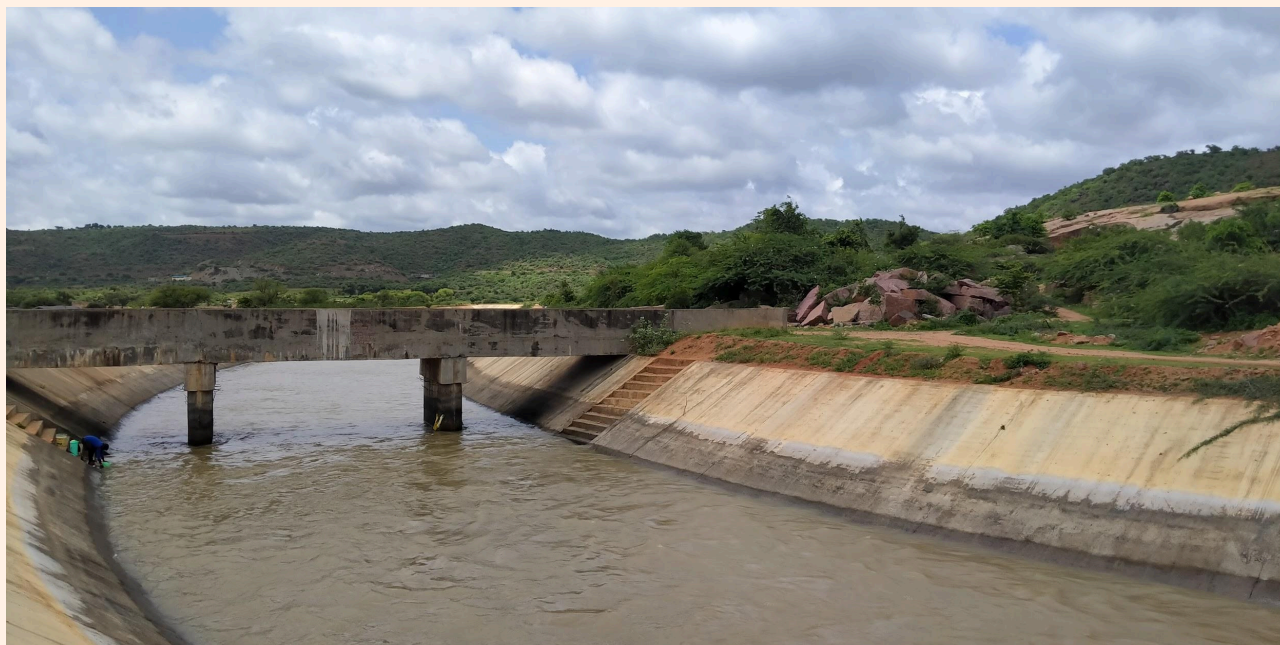
Figure 11: Narayanpur Right Bank Canal
