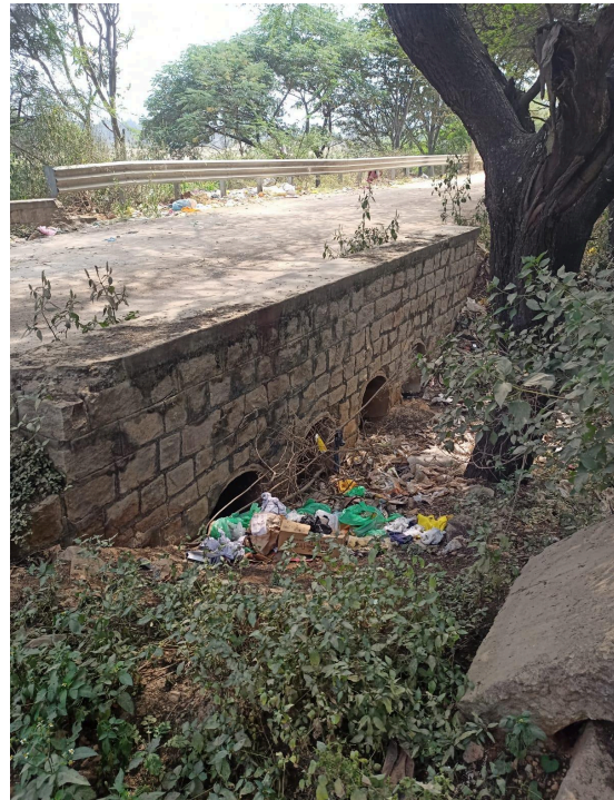
Figure 3.10: View of inlet 2
